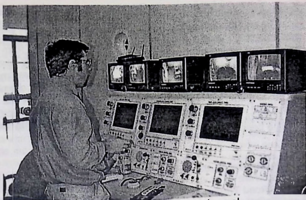
A close up of the control panel
